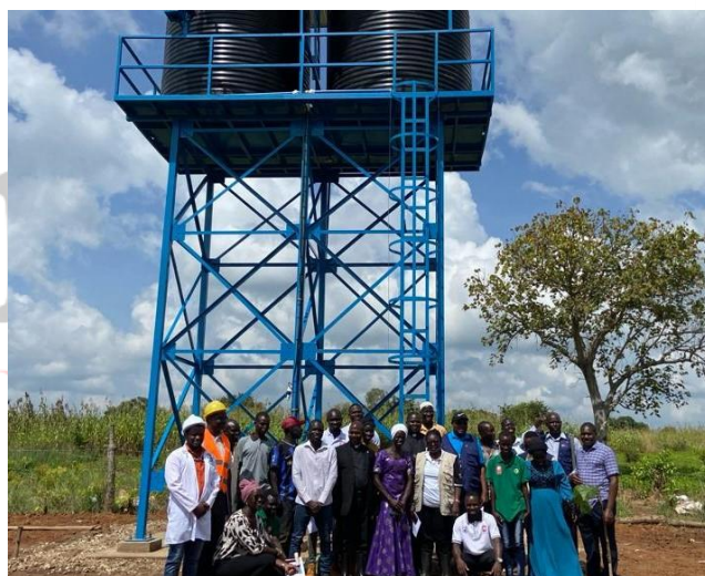
Inspection of the hybrid power water system constructed to provide water through the irrigation system at Orchogandi farm in Yumbe district.
